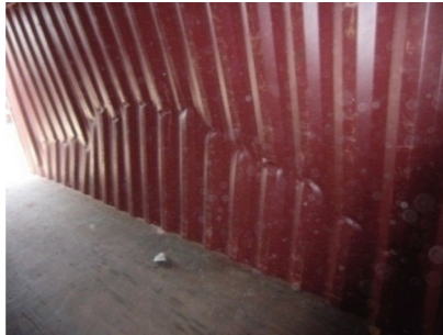
Figure 7.50 Damaged CTU side wall
