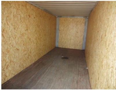
Figure 7.53 Lining a 40-foot container with chipboard panels
