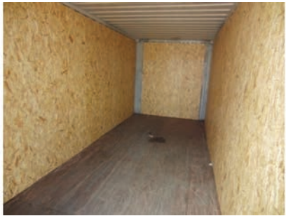
Figure 7.53 Lining a 40-foot container with chipboard panels
